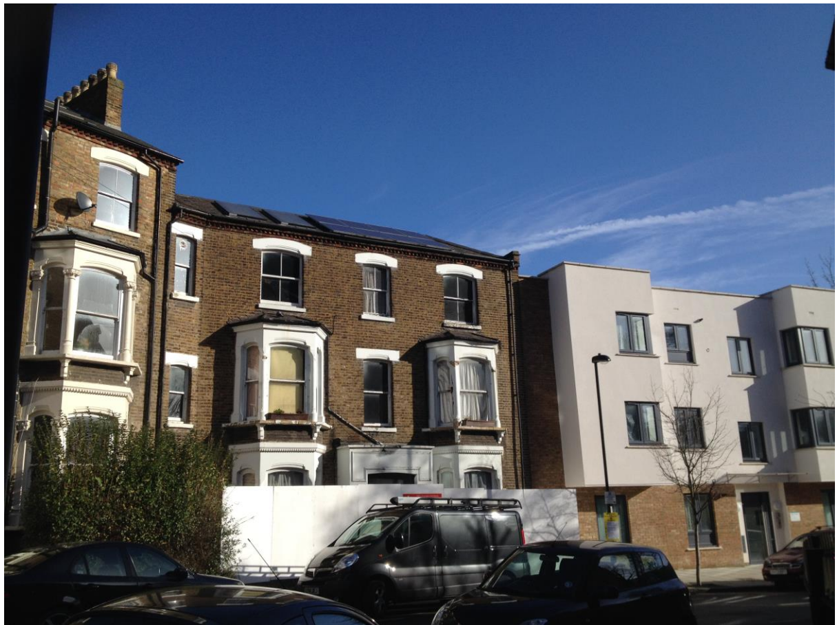
Image 4. – View of from elevation from Tremlett Grove
