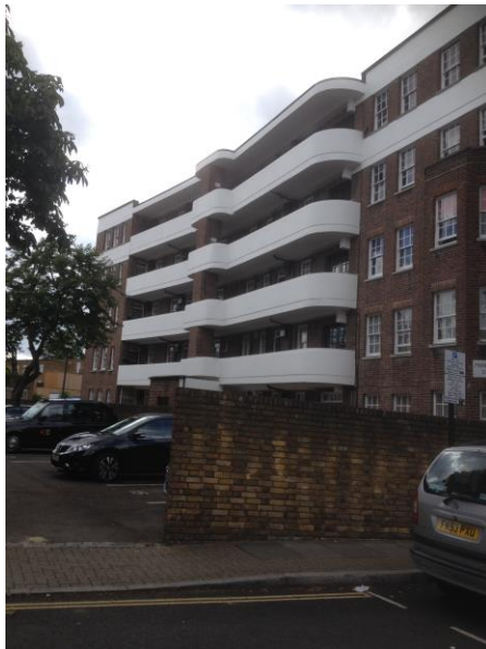
Image 2: View into the site.
